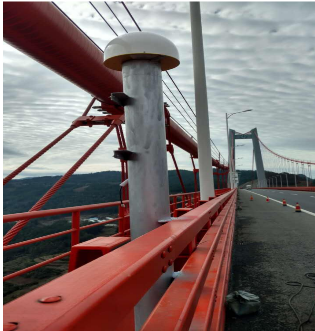
Fig. 8 Application of BDS-Based Bridge Integrity Online Smart Monitoring System
