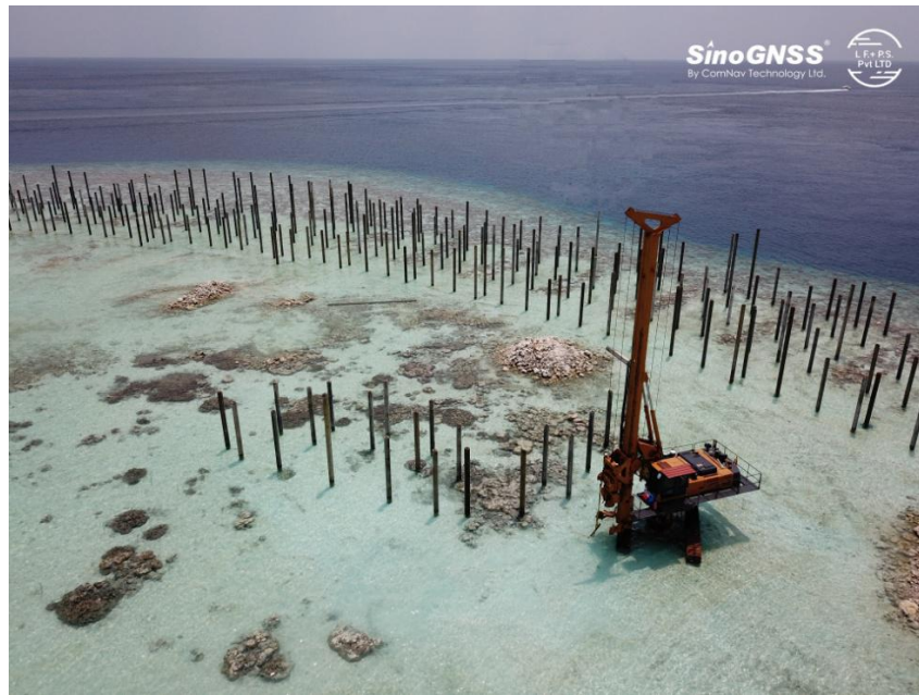
Fig. 29 BDS High-precision Receivers Used for Maldives Offshore Piling
