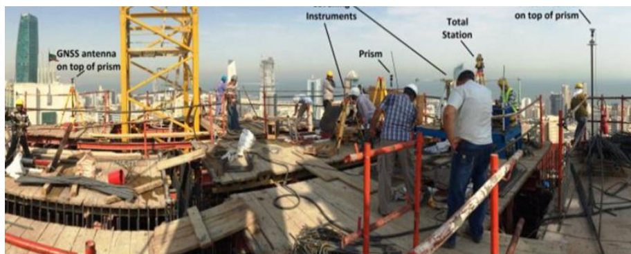
Fig. 26 BDS High-precision Receivers Used for Constructing the Headquarters Building for the National Bank of Kuwait
