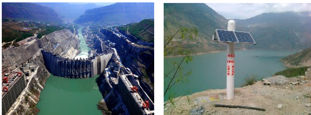
Fig. 13 BDS Hydroelectric Dam Deformation Monitoring
