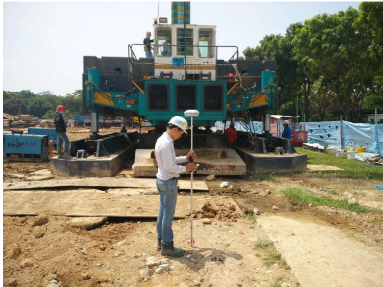
Fig. 30 BDS High-precision Receivers Used for Piling in Singapore
