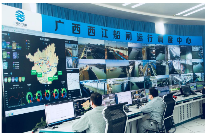
Figure 7 Guangxi Xijiang Ship Lock Operation and Scheduling Center
